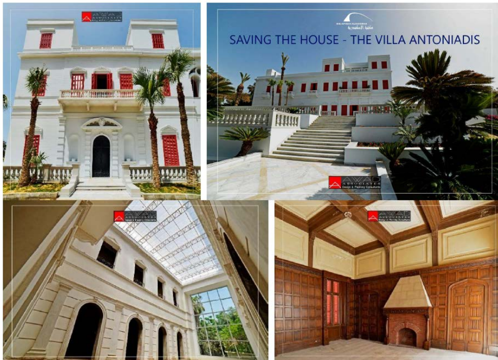
Figure 5: The Villa after renovation (Khalil, Hammouda, and El-Deeb 2018).
