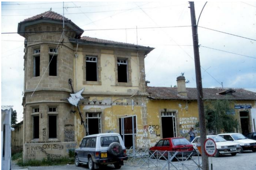
Main façade of the pilot case study building.
