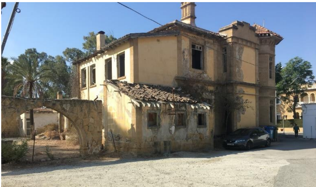
North-East façade of the pilot case study building.
