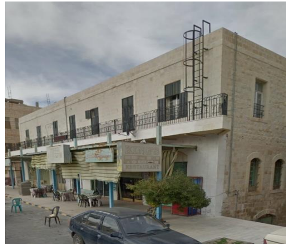
New façade of the pilot building: front view
