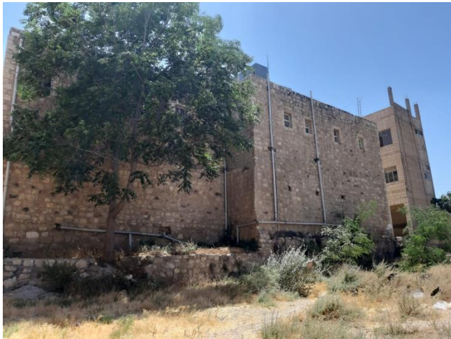
Old façade of the pilot building: back view
