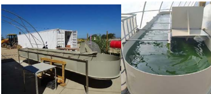
Figure 148. Microalgae cultivation plant during installation (left) and after operation (the reactor with the microalgae; right) in the salina Preciosa and Roqueta, Cádiz, Spain. ©H.Clavero (left) and Marambay (right)
