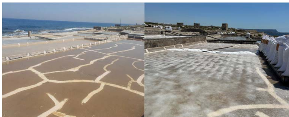
Figure 160. Salt ponds rehabilitation (left). Salt production in rehabilitated salt ponds (right), Blanc Sel Salinas, Anfeh, Lebanon. ©Jessica Najjar/Blanc Sel Salinas
