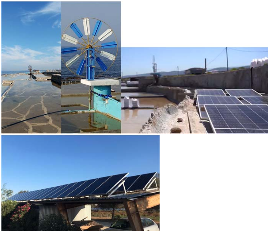
Figure 17. Traditional windmill restored (top, left), now running with a solar energy-powered pump; and solar panels being installed in the salina (top, right), Sleiman Salinas (Anfeh, Lebanon; MedArtSal project actions). Installation of solar panels (36 in total) on the roof of the car park in Salinas de Chiclana, Spain (below). ©MedArtSal project (above) and Salinas de Chiclana (below)
