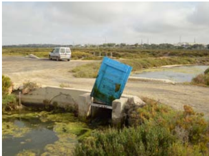
Figure 4. One of the gates controlling the flow of water in Salina La Esperanza (Cádiz, Spain). ©Yana Korneeva Abdulaeva
