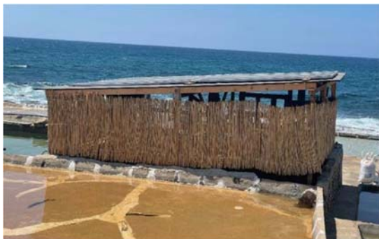
Figure 164. Installation of solar panels on the roof of the hut in the salina. ©Georges Sleiman/Evaura
