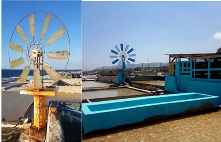
Figure 165. The windmill, a characteristic feature of these saltworks and a tourist attraction, before its restoration (left) and once restored for water pumping, next to the spa pool (right). ©Georges Sleiman/Evaora
