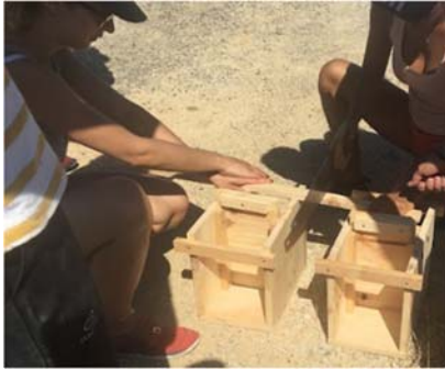
Figure 93. Building of salt pan wood gates by workshop participants. ©SC-ISE. UCA
