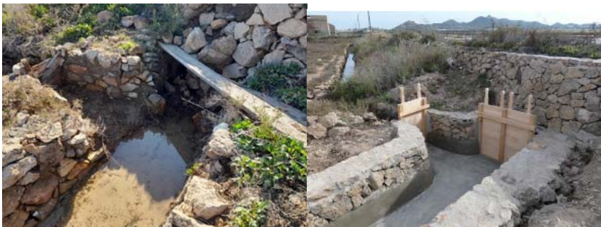
Figure 146. The sluice gates before and after the reconstruction. ©ANSE
