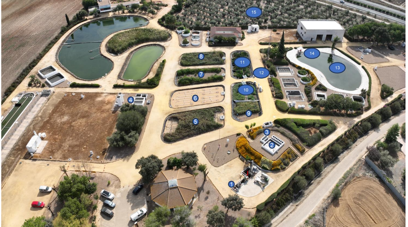
Figure 11. Aerial view of treatment units at Carrión de los Céspedes Experimental Center, Seville, Spain: 1- Pre-treatment; 2- Homogenization tank; 3- Distribution channels; 4- Imhoff Tank; 5- Vertical Subsurface CW-1; 6- Vertical Subsurface CW-2; 7- Vertical Subsurface CW-3; 8- Free Water Surface CW; 9- Horizontal Subsurface CW; 10- Aerated vertical-horizontal CW; 11- Floating helophytes; 12- reception and distribution chamber; 13- Storage pond; 14- Post-treatment: ultrasound unit + automatic pressure sand filter + manual cleaning mesh filter + pressure group; 15- Olive grove plot.
