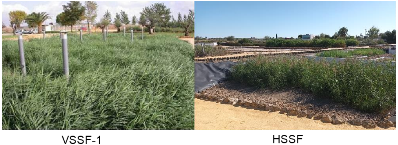
Figure 5. General overview of the Vertical Subsurface (VSSF-1) and Horizontal Subsurface (HSSF) flow Constructed Wetlands
