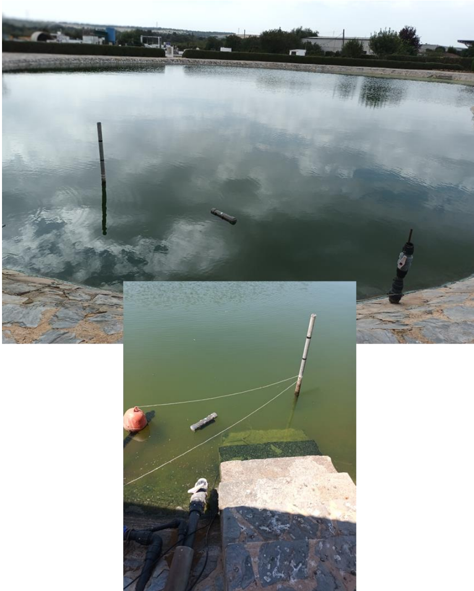
Figure 12. General view of the ultrasound equipment installed in the storage pond.
