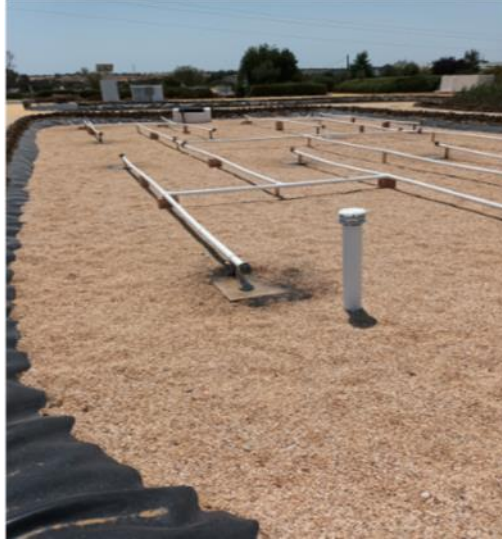
Figure 7. General overview of the Vertical Subsurface Flow (VSSF-2) Constructed Wetland
