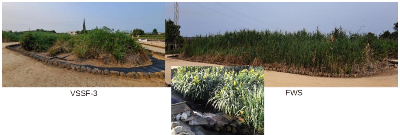
Figure 6. General overview of the Vertical Subsurface (VSSF-3) and Free Water Surface (FWS) Flow Constructed Wetlands
