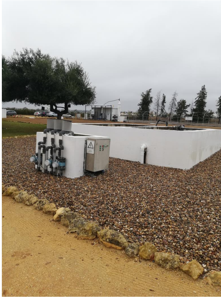
Figure 4. General overview of the Imhoff Tank
