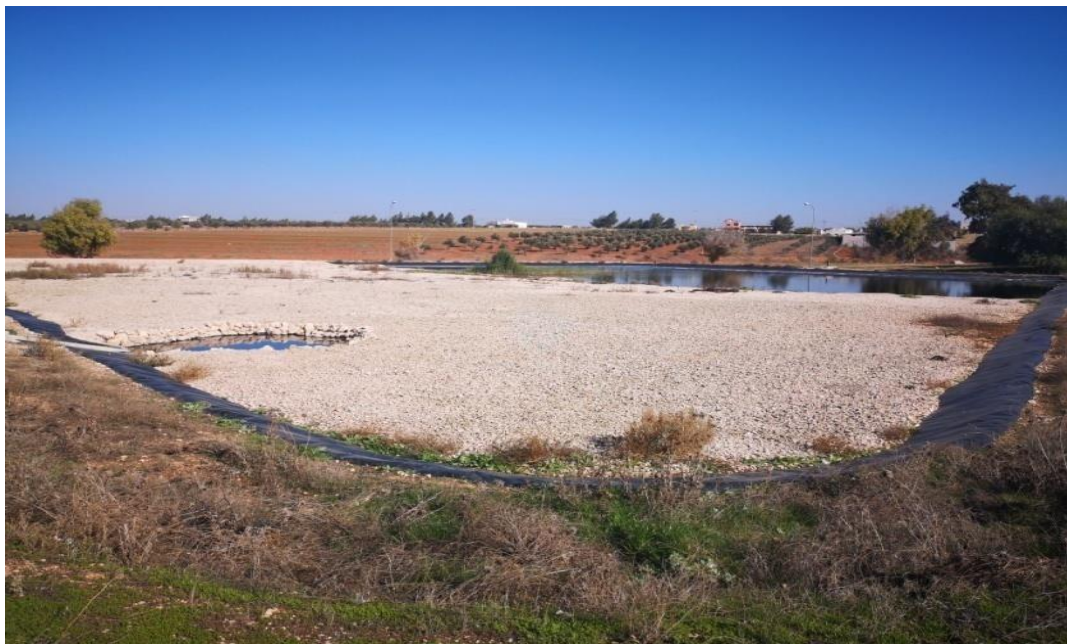
Figure 9. Overview of the Rock Filter for microalgae removal
