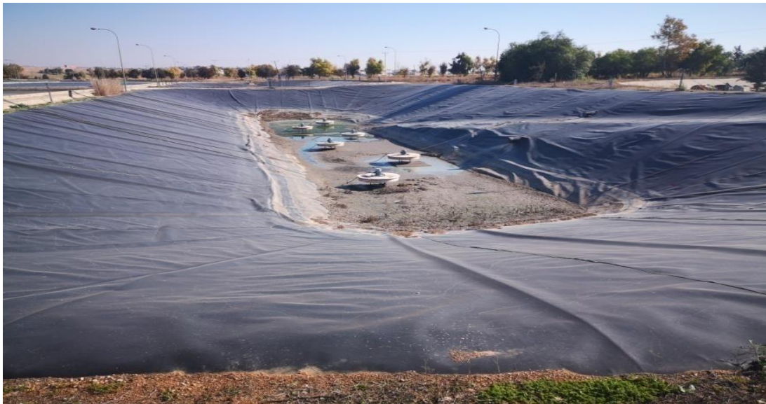
Figure 5. Overview of one of the two Equalization Ponds
