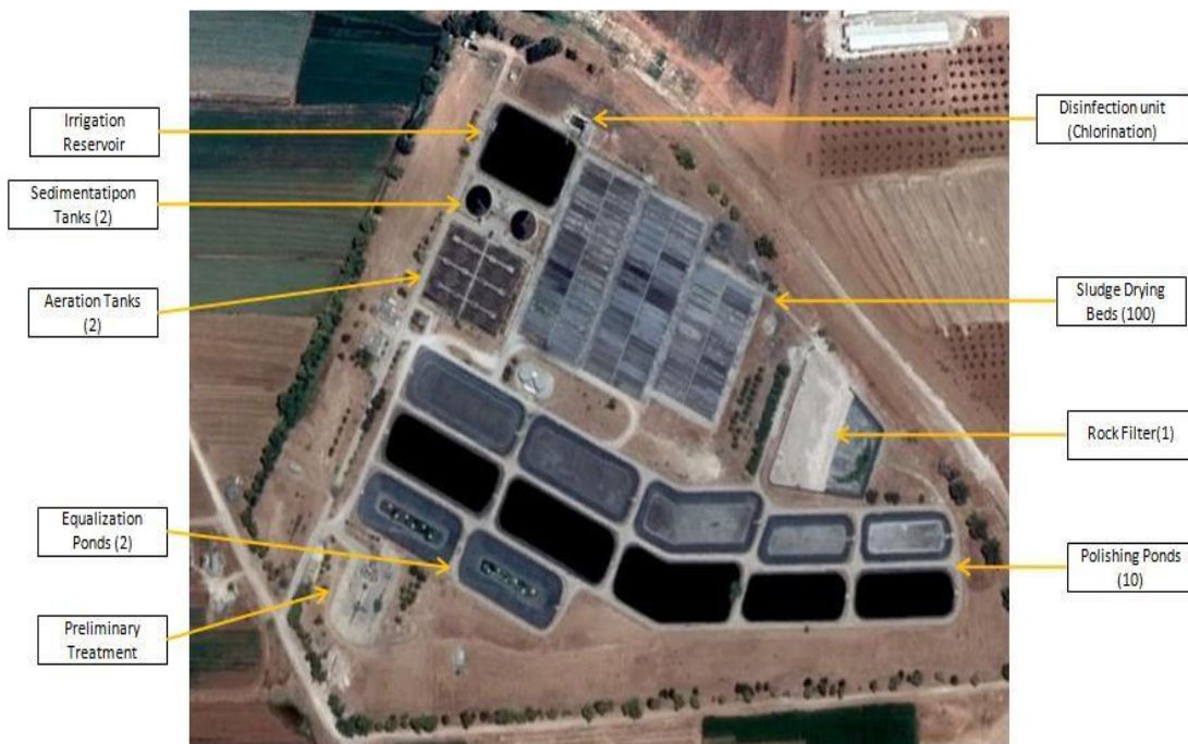
Figure 3. Overview of Ramtha WWTP, including treatment units
