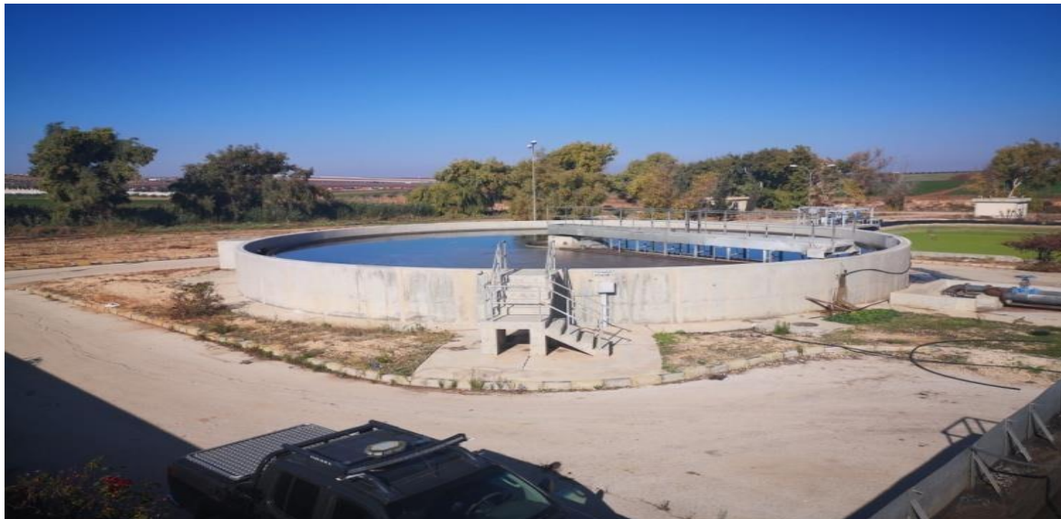
Figure 7. Overview of one of the two Sedimentation Tanks
