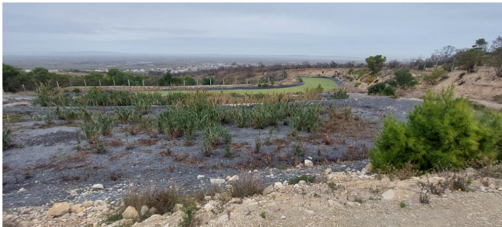
Figure 14. The constructed wetlands CWs
