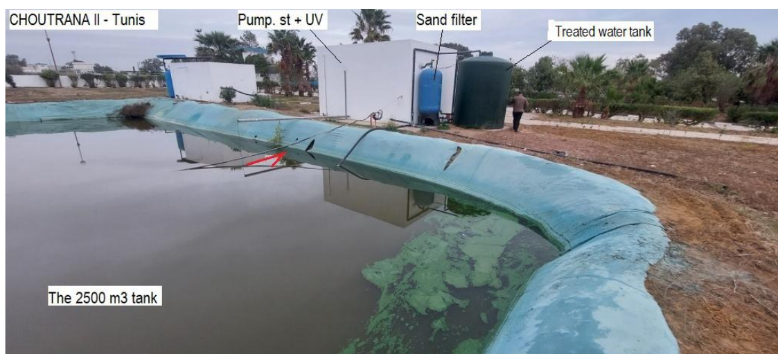
Figure 8. View of the existing 2500 m 3 tank in the Choutrana II WWTP
