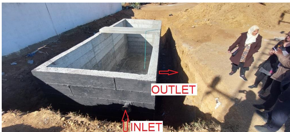
Figure 16. The RCC tank
