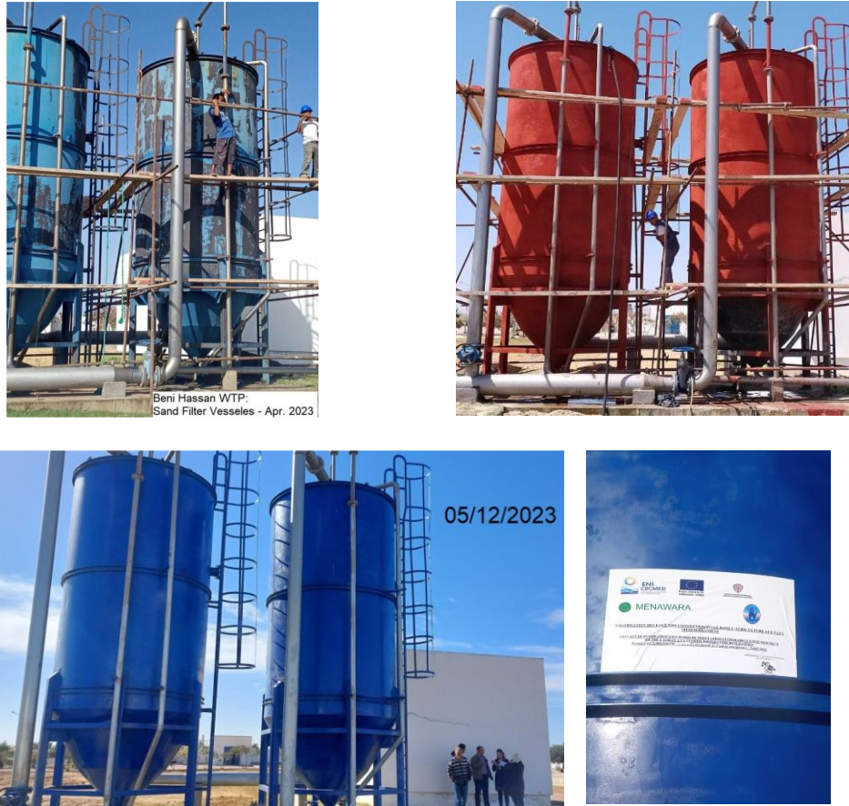
Figure 16. Sand filter, relining of the steel vessels
