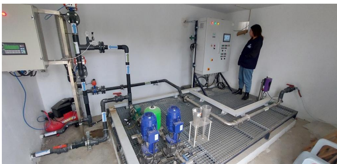
Figure 10. Overview of the pumping station
