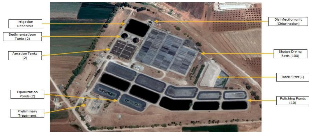
Figure 2: Overview of Ramtha WWTP, including treatment units
