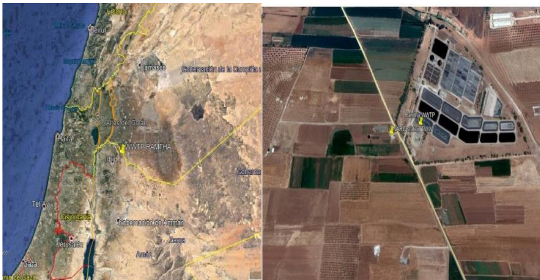
Figure 3. Location of Ramtha WWTP and Treated Wastewater Research Station, in Jordan.
