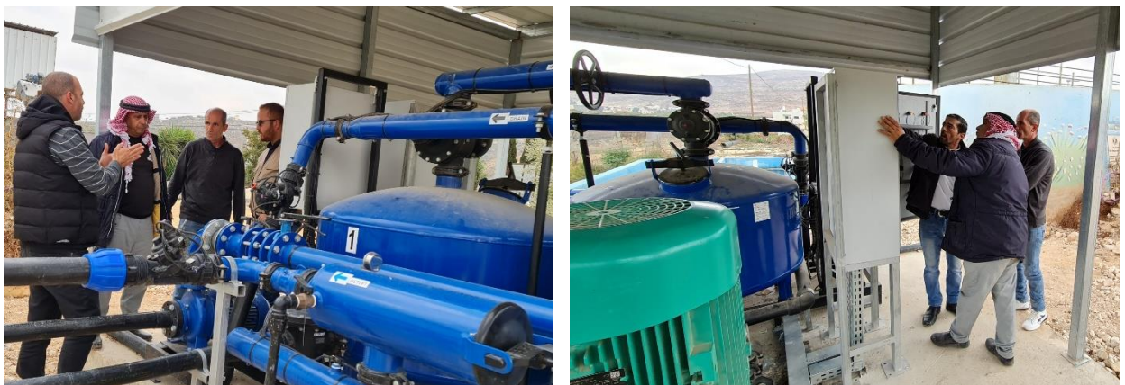
Figure 4. Training on operation and maintenance of the 2 installed pressured sand filters.
