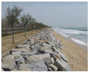
Figure 11. Protection structure parallel to the coast made of stones in Spain El Masnou (After the works).
